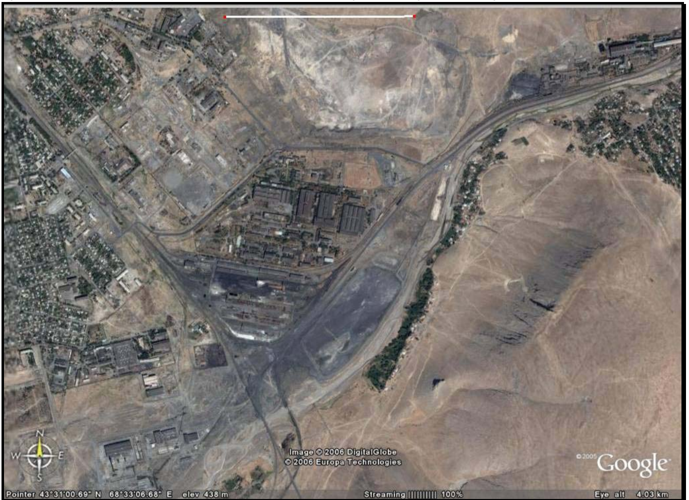
Figure H.16. Kentau. Major areas of derelict and despoiled land due to heavy metal mining and processing. Scalebar 1km.
